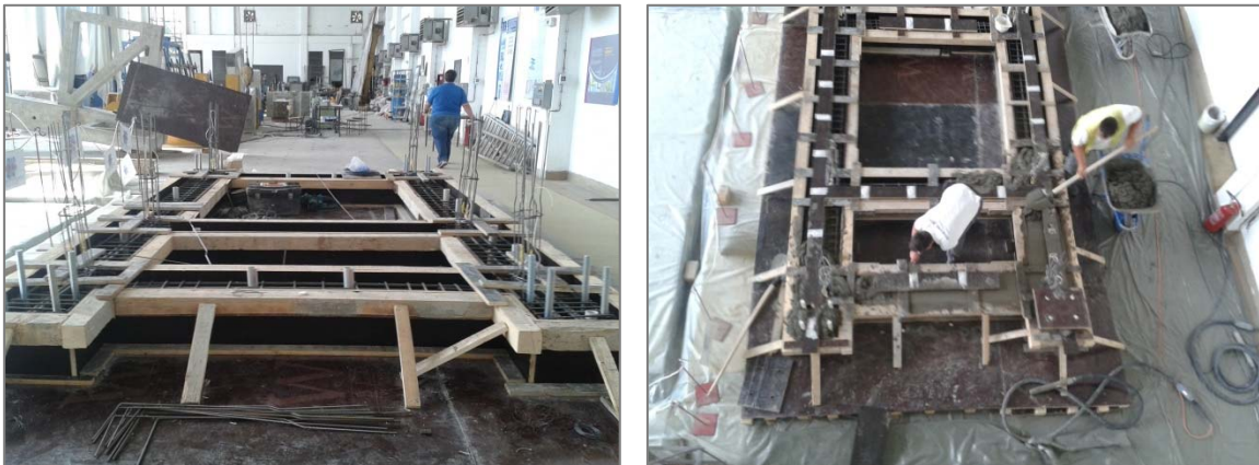
Figure 4.18 Construction of RC foundation of the scaled model
