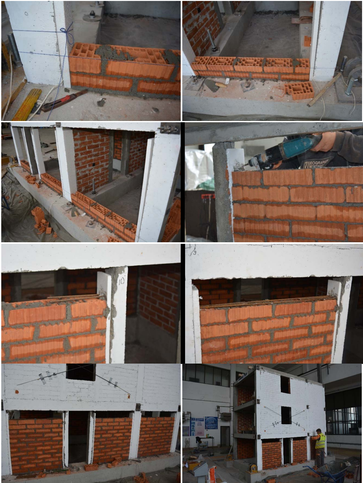
Figure 4.21 Construction of the Model IW-SB – variant solution b)
