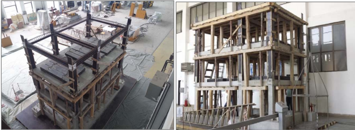
Figure 4.19 Construction of the RC frame of Model IW-SB
