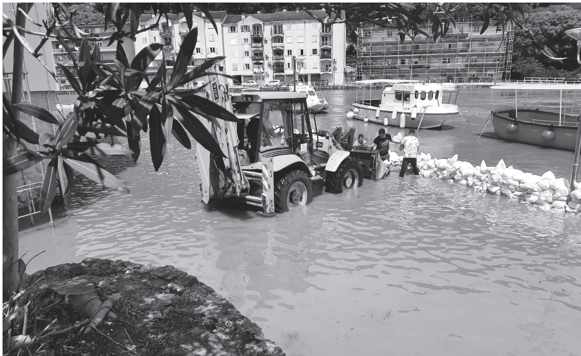
Figure 4. Flood in Obrovac (May 2023) (photographed by I. Peša)
