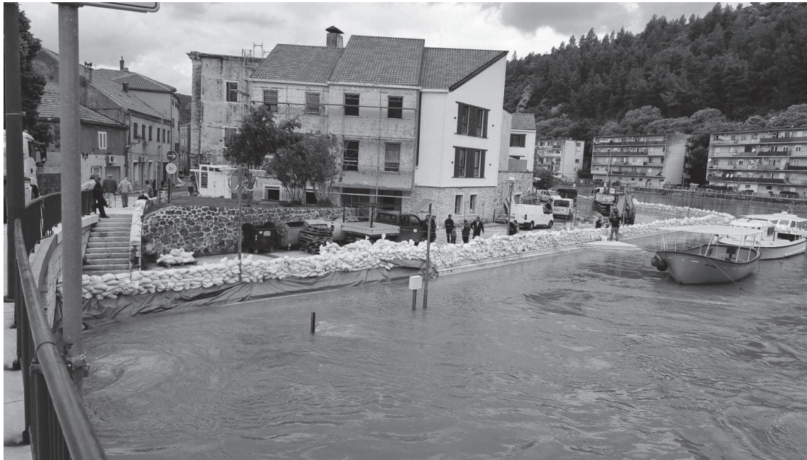
Figure 3. Flood protection on the left bank of Zrmanja in Obrovac (May 2023) (photographed by I. Peša)
