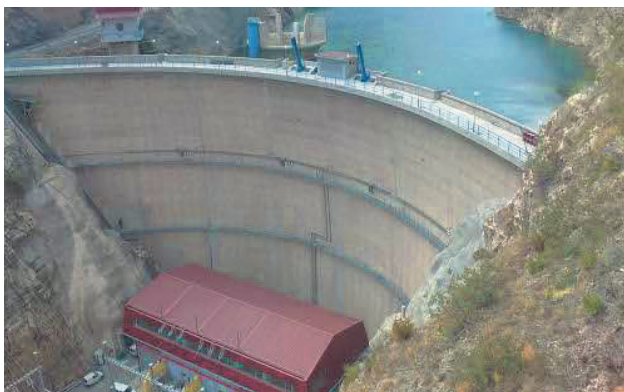
Figure 21. Arch dam “Sveta Petka” on the river Treska (construction completed in 2012) ( https://mk.wikipedia.org/wiki/HEC_Sveta_Petka ).
