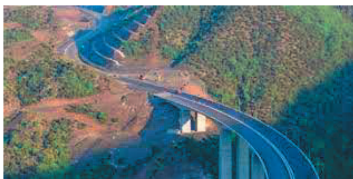
Figure 24. Some structures at highway E-75, section from Demir kapija to Smokvica (cut is in diabases with a height of about 70 meters).
