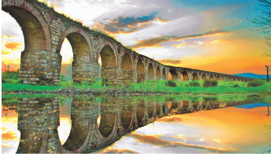
Figure 1 View on the Skopje Aqueduct
