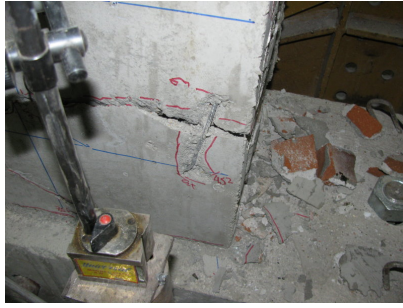
(a) Toe cracking and bending of horizontal reinforcement
