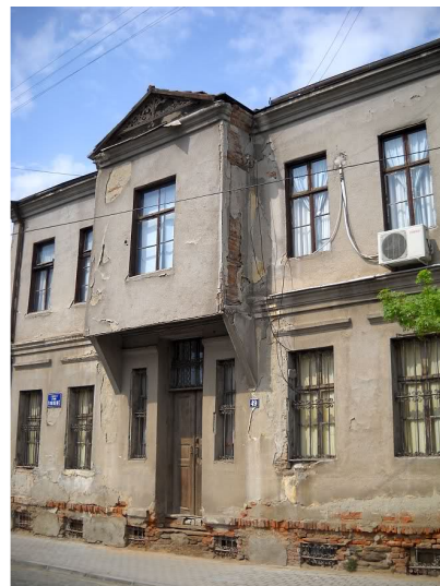
(a) URM building with bricks on both floors (Madzir Maalo)
