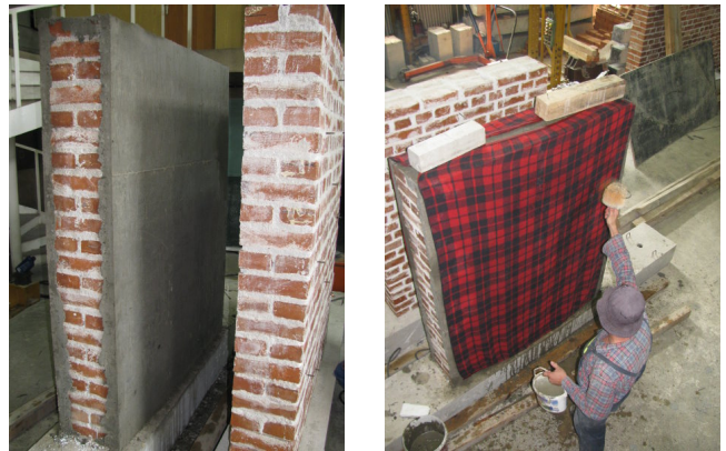
(a) SMW after removal of the moulds (b) Protection of a wall with wet blankets on both sides
