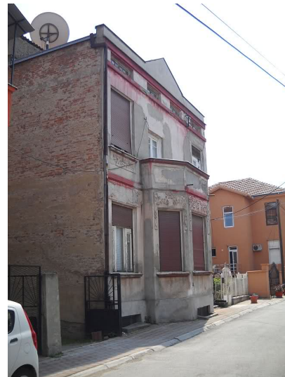
(b) URM building with RC floors (Debar Maalo)
