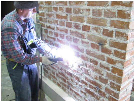
(a) Welding of reinforcement bar pieces over the anchors
