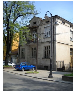
(b) Brick masonry house in Skopje
