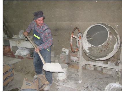
(a) Preparation of concrete for the jackets
