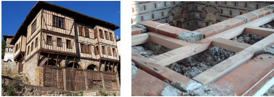
(a) Wood cantilever extension at house in village Vevchani (b) Wood truss 'santrach' on double wythe wall
