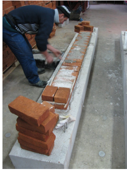
(a) Laying of the first course of bricks
