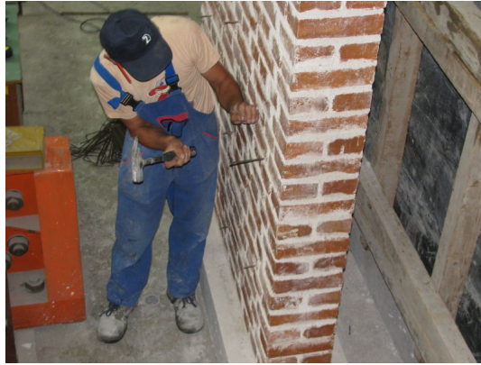
(b) Hammering anchors into UMW
