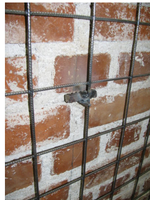
(b) Close-up view of welded reinforcement bar over anchors and welded wire-mesh to anchors
