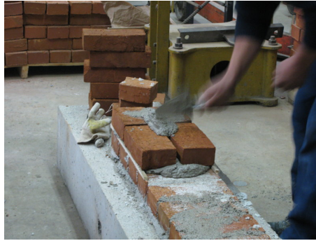
(b) Laying the second course of bricks and filling the head joints with mortar
