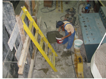
(b) Transport of fresh concrete
