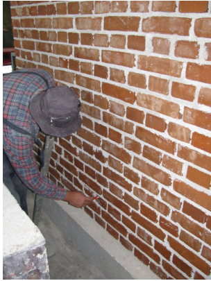
(a) Marking locations for connecting anchors
