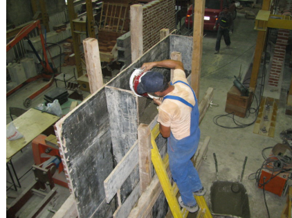
(c) Casting of concrete into moulds
