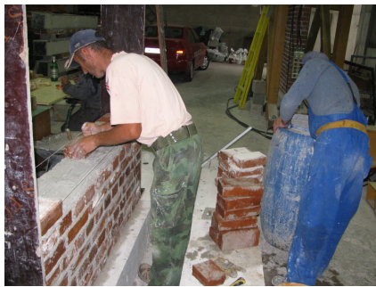
(a) Soaking of the bricks before construction
