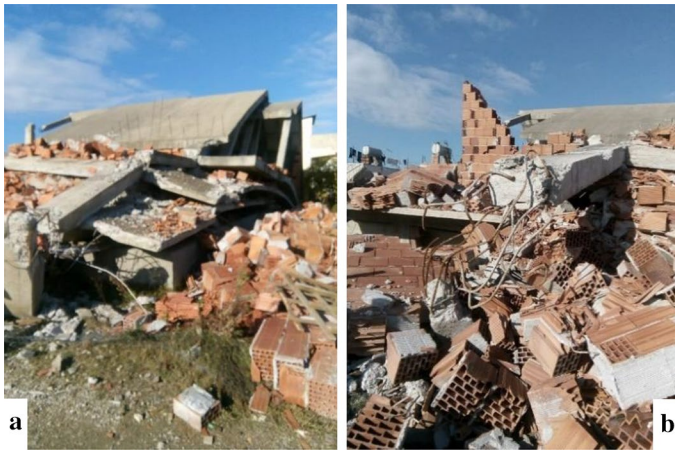
Fig. 23 Residential structures in the phase of construction that collapsed under the effect of the earthquake (Grade 5). Flat slab system where tiles and stirrups are with small diameter and stirrups located in long distance
