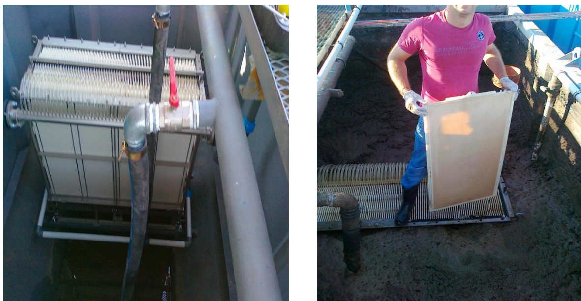
Figure 1. Submerged MBR module with PVDF membranes
