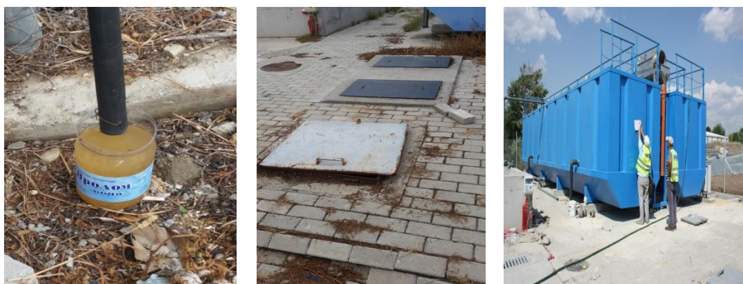
Figure 2. Wastewater sample and sample point before the MBR Plant
