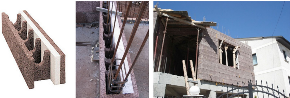
Figure 8. a) Hollow wood-chip concrete blocks with integrated insulation; b) Hollow wood-chip concrete blocks - placing reinforcement in the wall; c) Hollow wood-chip concrete blocks – mounting elements.
