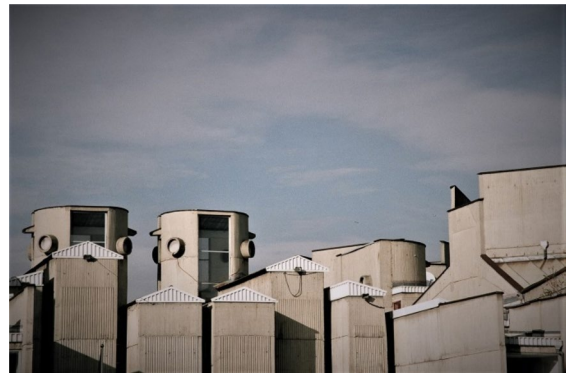
Img14_Brutalizam in function of UKIM Milosavljevska Vesna
