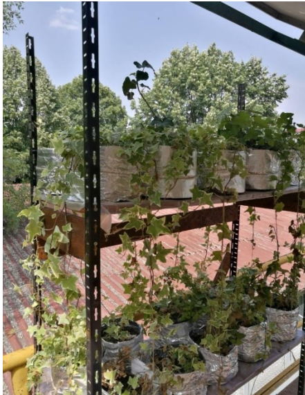
Fig.2. The green wall structure
