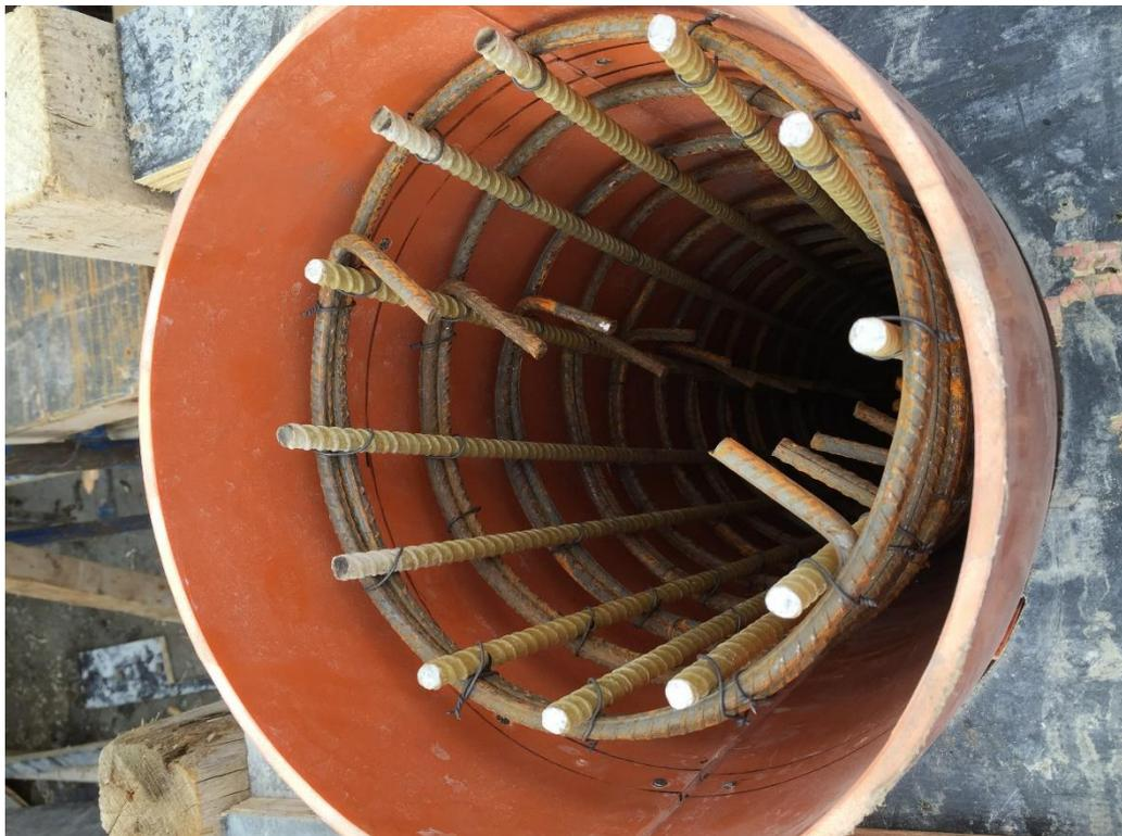
*Figure 5 - Reinforcement of Columns – Longitudinal Rebars GFRP – Stirrups 7.5cm spacing*
