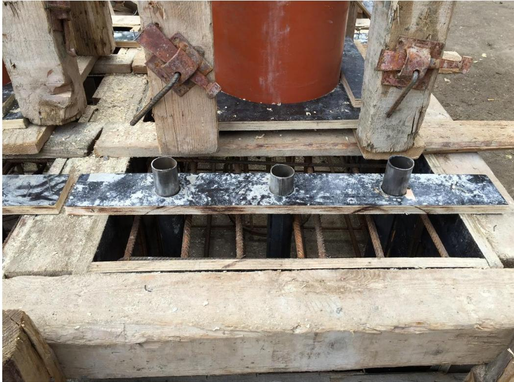
*Figure 6 - Placement of Steel Pipes for fixing of anchors in foundation*
