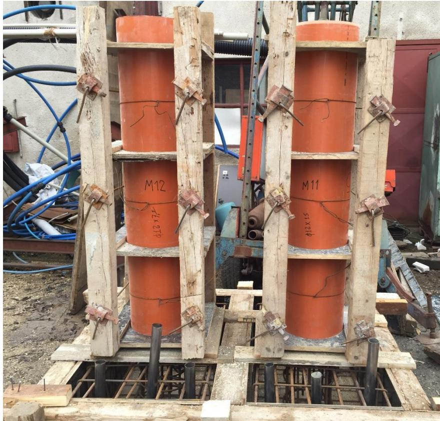
*Figure 3 - Formwork of Columns and Reinforcement of Columns*
