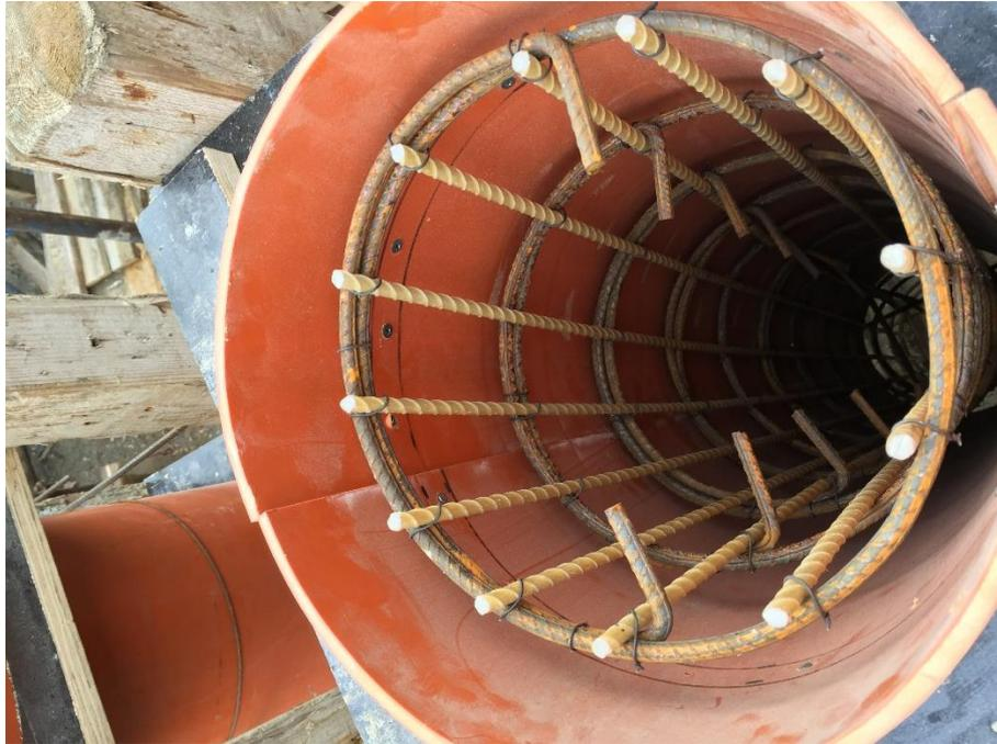
*Figure 4 - Reinforcement of Columns – Longitudinal Rebars GFRP – Stirrups 15cm spacing*
