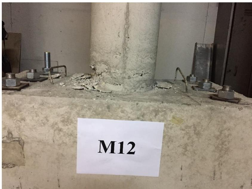
*Figure 8 - Column M12 – Cover spalling*
