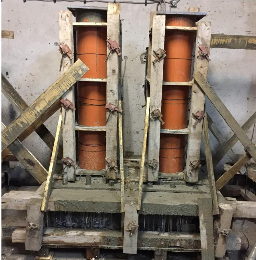
*Figure 8 - Concrete columns after concreting*
