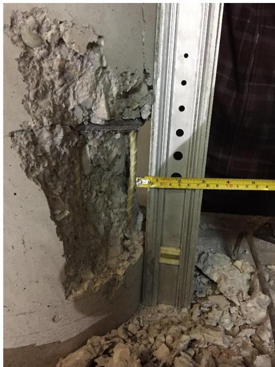
*Figure 22 - Column M31 – Different cover in left and right side of column*
