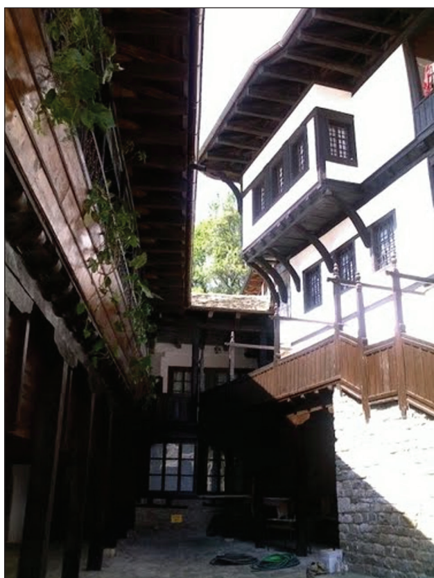
Figure 17. The brave construction solution with a console expanding of the flooring and the staircase part makes this architectonic element unique and unrepeated. The supporter is repeated in the same form and by supporting the angle from the extremely expanded eave so that the builder creates a visual ending of the building.
