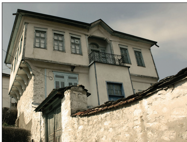
Figure 11. Cantilevered differentiation at the top floor which continues the line of the street facade is enriched with baroque forms at the vertical supporters.
