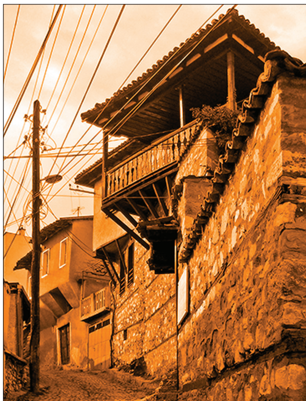
Figure 14. Typical example of triangle cantilevers. A strong contrast on the rustic surface of the wall made of stone and the white surface on the upper floors. A logical position of the supporters which changes the angle of transmission of the load. [4]
