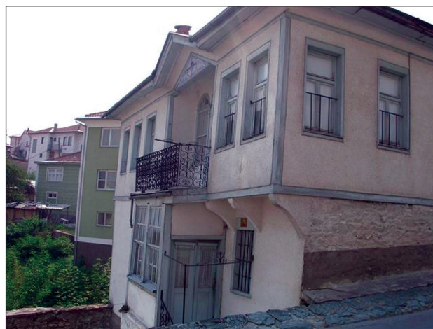
Figure 9. Characteristic example of a Krushevo house with broken and asymmetrical geometric form at the ground floor is accomplished and flattened at the floor by using the cantilever, that way forming also a porch. The characteristic and conspicuous tympanum on the roof, the top open balcony at the floor disturbs the harmony of the rhythm of the windows aperture.
