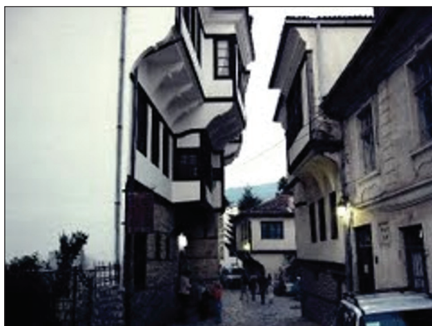
Figure 5. What the cantilever is with its qualities for the construction that is the construction for the narrow path. The passer-by has perfect views towards the architecture and the sky.
