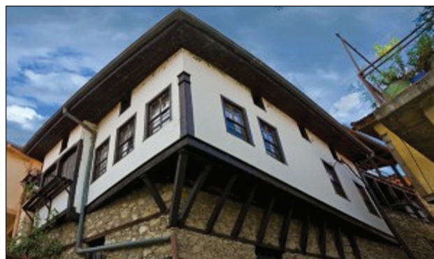
Figure 15. The asymmetrical base of the ground floor, dictated by urban and terrain conditions, is straightened on the upper floors by expanding the triangle cantilevers in order to create standard rooms and a terrace.
