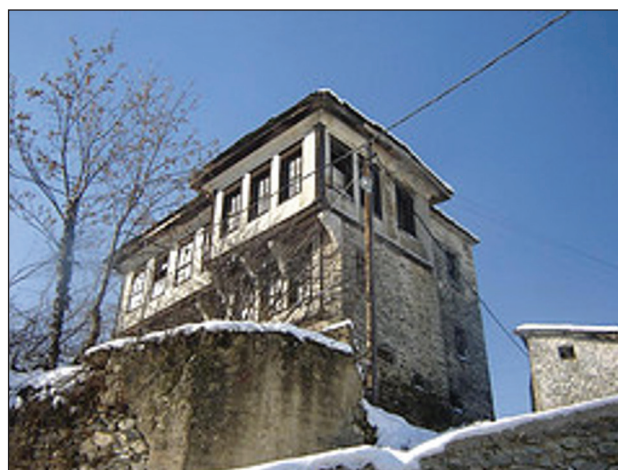
Figure 10. Cantilevers with curving baroque forms exposing the floors, forming dynamic housing facility as a contrast to the harmonic rhythm of the windows and the simplicity of the stone walls. The traditional compatibility of the blue color on the stone, the white one on the stony walls and the dark color on the window frames made of wood is present.
